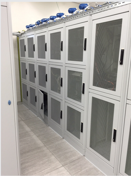
A look at the racks housing PROMISE FileCruiser at ICTeam, providing its customers with a private file synchronization and sharing solution.
